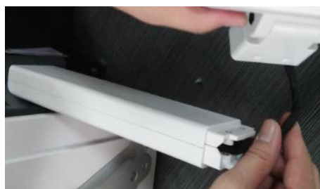
⑧ Insert additional cables to the rod
